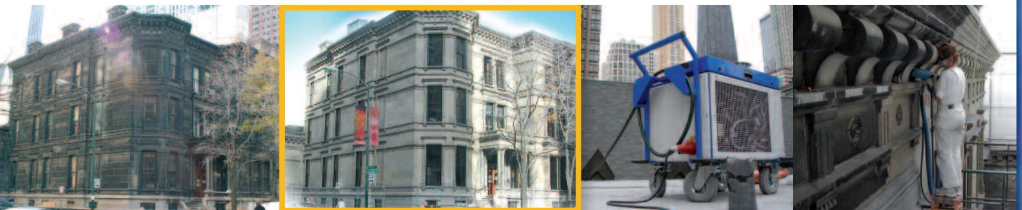
Chicago-City: Restoration of a natural stone mansion built in 1883, worldwide first big size restoration totally and only proceeded with laser technology, ca. 2500 m 2 surface
